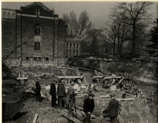
Photographer: Unknown Construction of Emmanuel College, 1930 1991.161/547 Victoria University Archives
